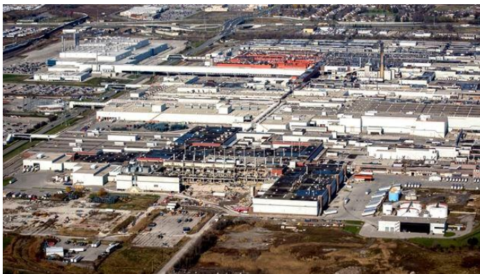
GM South Plant, Oshawa, Ontario
